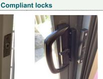
Door can be unlocked from Sliding door can be the inside without a key and unlocked from the inside locked / unlocked from the outside with a key. Sliding door can be unlocked from the inside without a key and locked / unlocked from the outside with a key.
