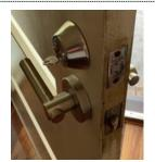
Only fitted door lock that needs a key to unlock the door from the inside and from the outside.
