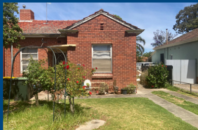
10 Kenilworth Ave, Edwardstown $395,000
